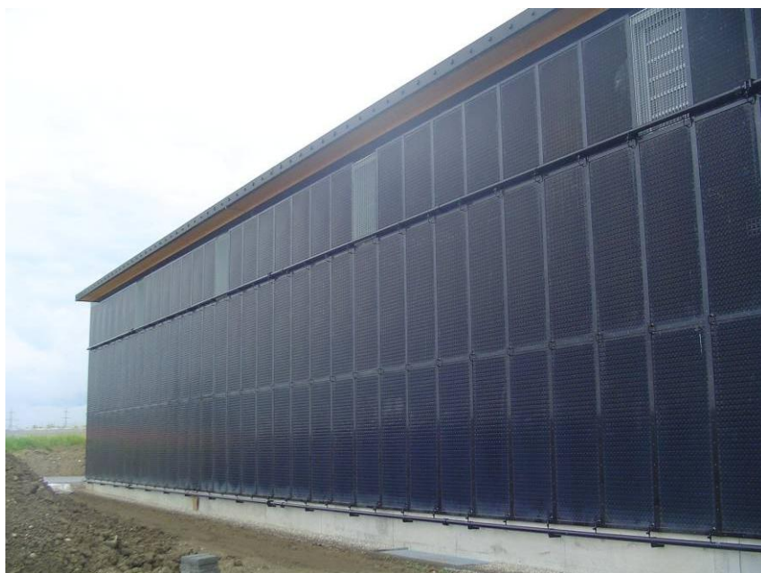
Solar thermal collector to supply heating- and warm water
