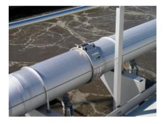
The movement will be guided into the coupling by using anchoring and guiding points for optimal axial movement compensation by STRAUB-FLEX. Correct anchoring and guiding points are requested
