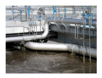
Joining prefabricated pipe elements connected with STRAUB-GRIP-L onsite
