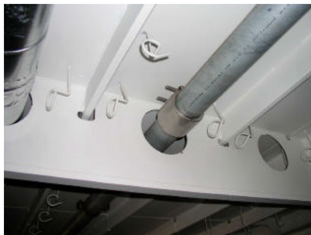
Minor requirements for structure leadthrough
