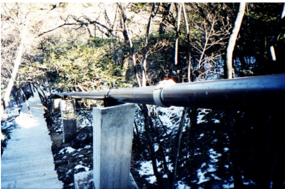
Pipe supported by concrete blocs (steepness approx. 100%)
