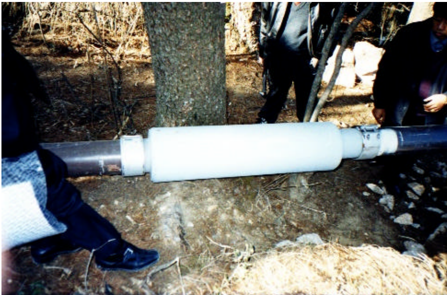
Installation of expansion joint with two STRAUB couplings.
